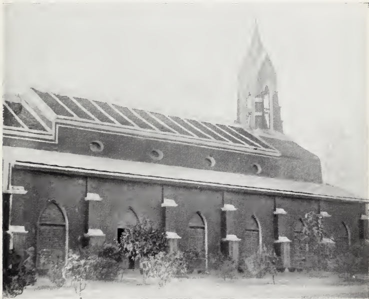
ST. PETER'S CHURCH, BIMLIPATAM.
